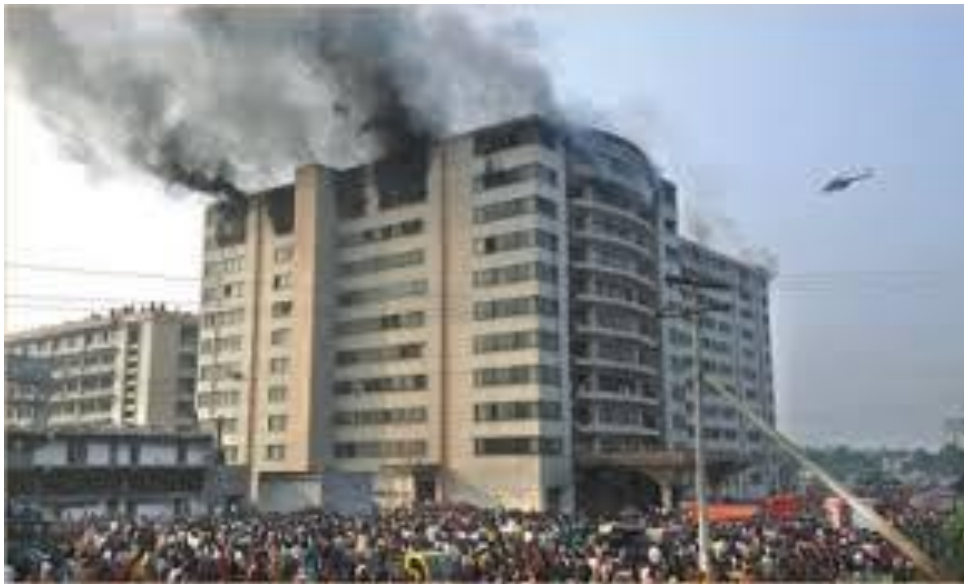
Fig 4.9- Ha-meem fire hazard
