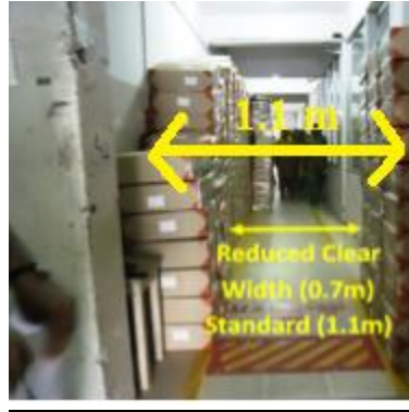
Fig2.1: Clear width of an exit corridor reduced by piled up boxes (Color figure online).
