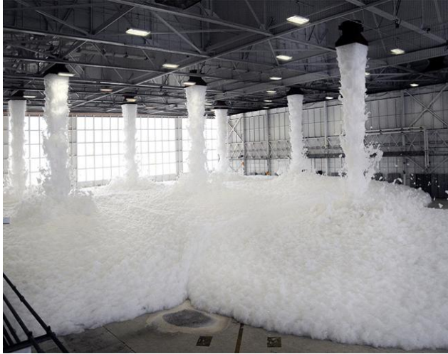
Fig 2.18: Foam extinguishing system
