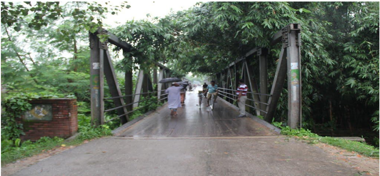
Figure 2.14: Truss with Steel Deck, Boalia Bazar, Nalchiti, Barisal
