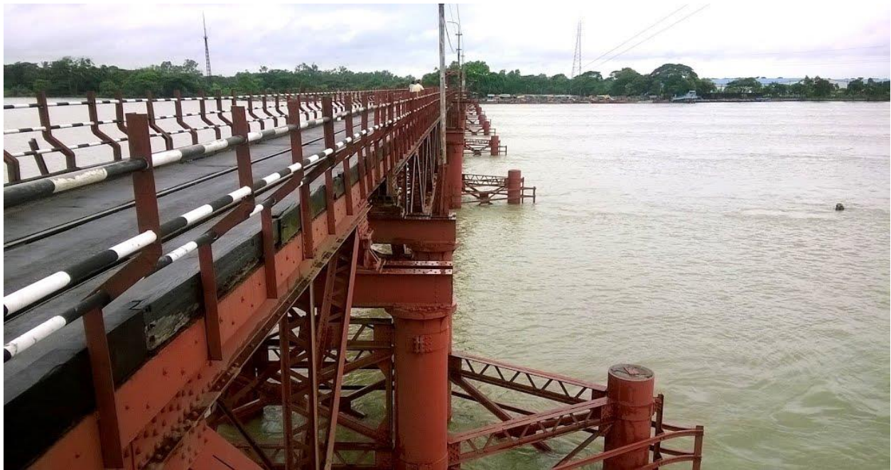
Figure 2.15: Bailey Bridge with Steel Deck, Kalurghat Bridge, Chittagong
