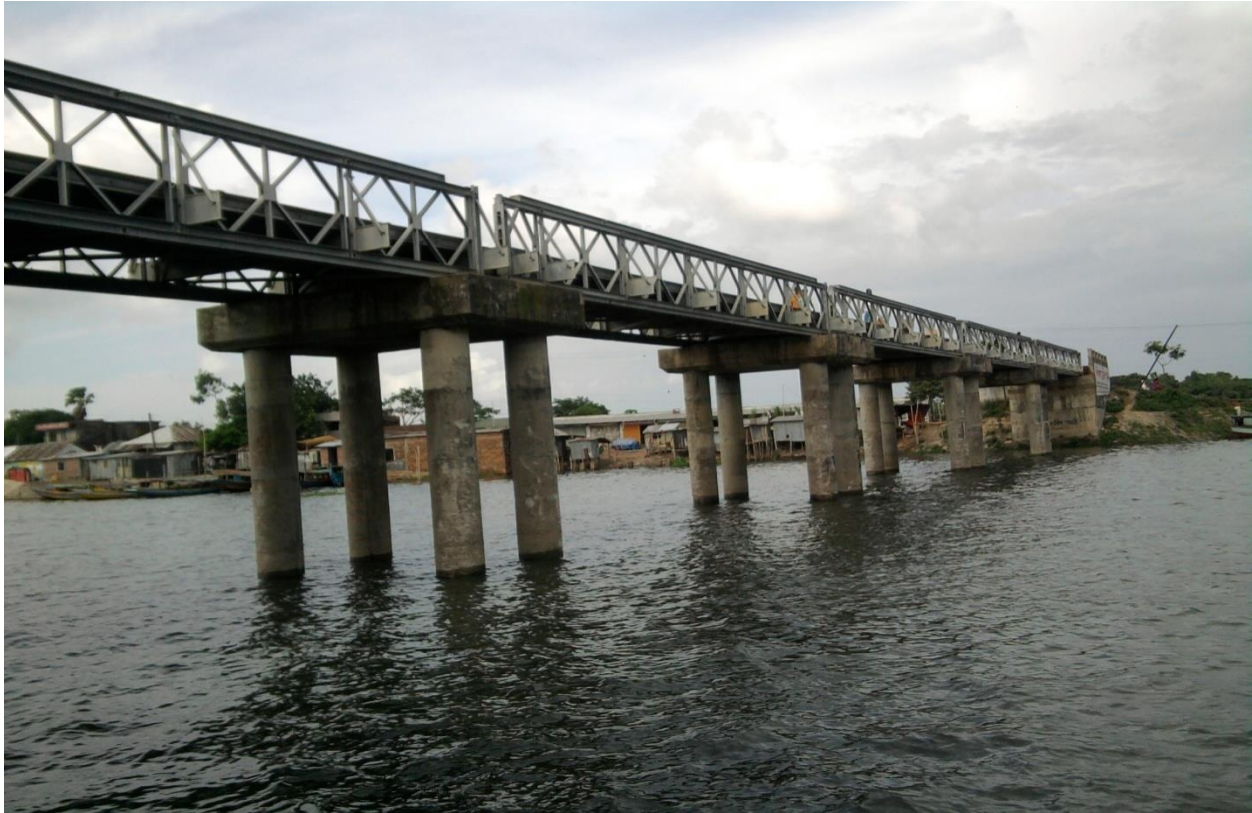
Figure 2.17: Steel Beam & Reinforced Cement Concrete (RCC) Slab, Isapur Bridge, Purbachal
