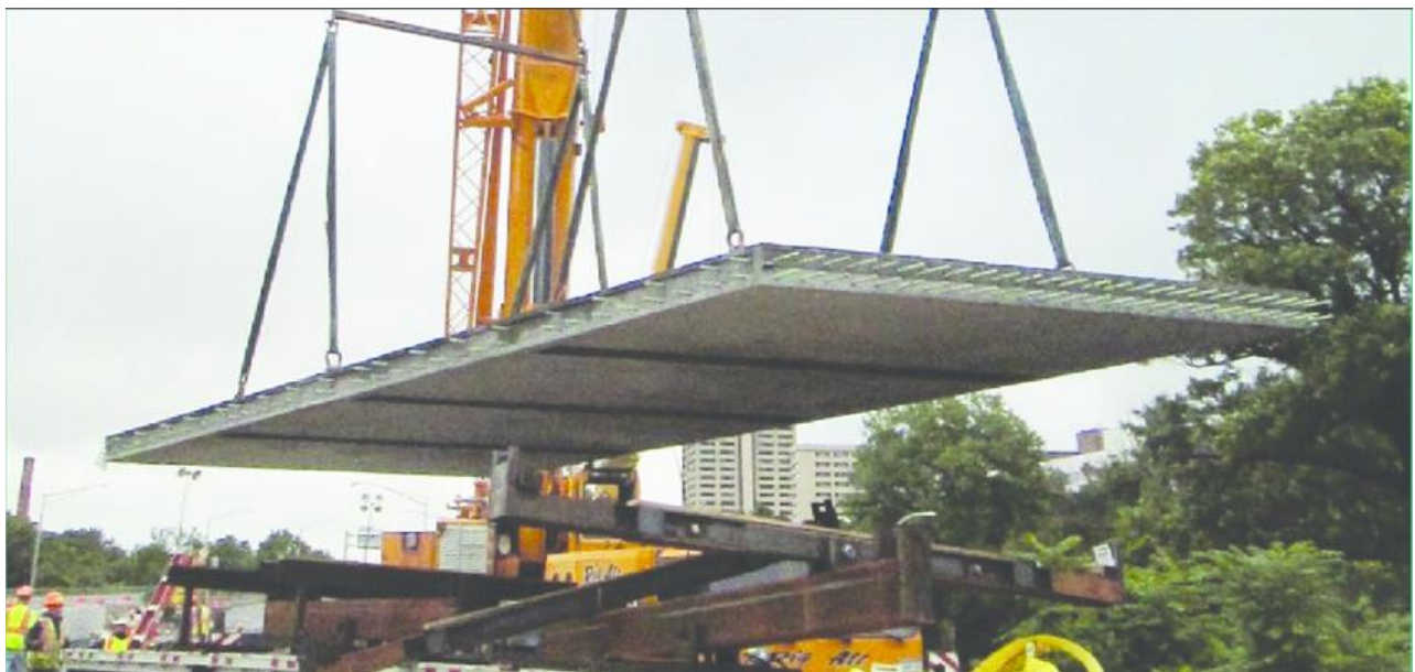
Figure 3.13: Placement of Deck Panel
