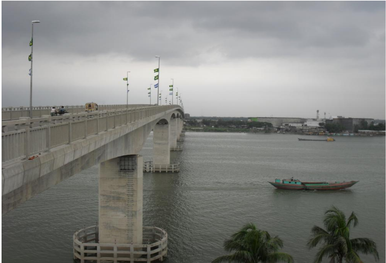
Figure 2.6: Reinforced Cement Concrete (RCC) Bridge, Dhaleswari River Bridge, Munshiganj
