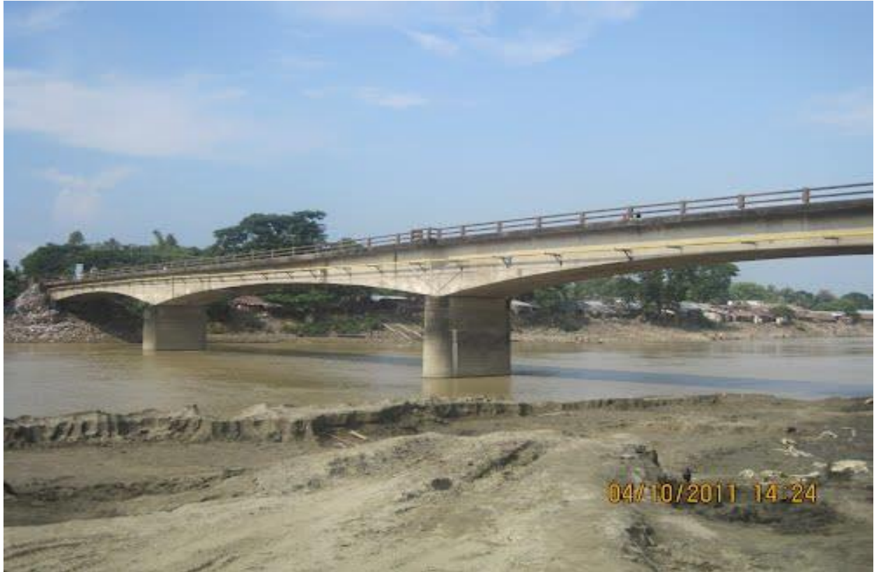
Figure 2.5: Reinforced Cement Concrete (RCC) Girder, Sangu Bridge, Bandarban
