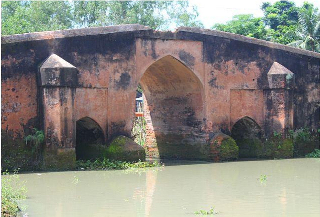
Figure 2.10: Arch Masonry, Mir Kadim Bridge, Munshiganj
