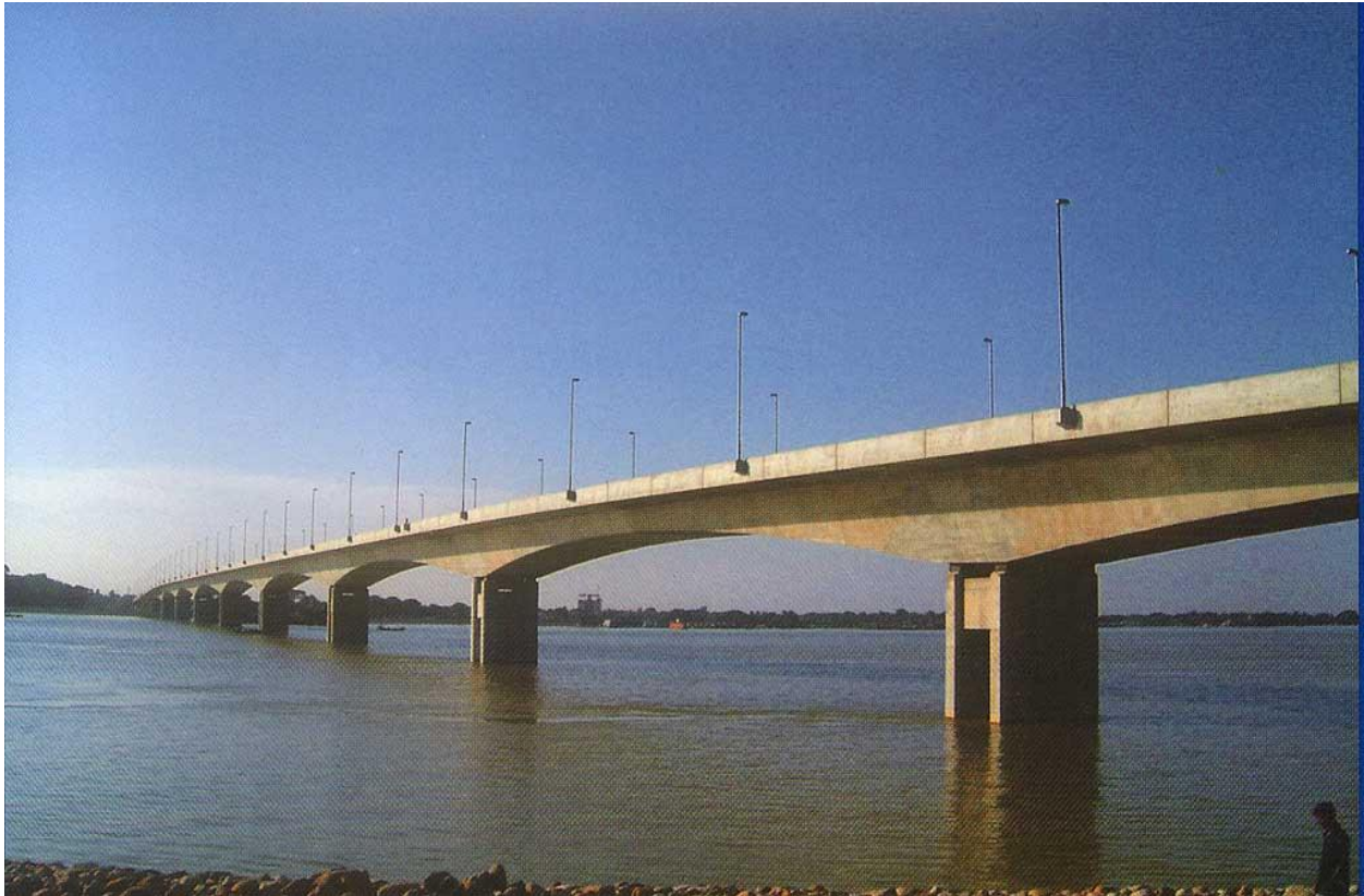
Figure 2.18: Pre-stressed Concrete (PC) Box Girder, Bhairab Bridge
