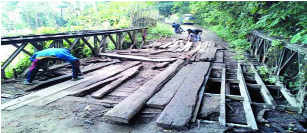
Figure 2.16: Bailey Bridge with Timber Deck, Koikhongjhiri, Bandarban
