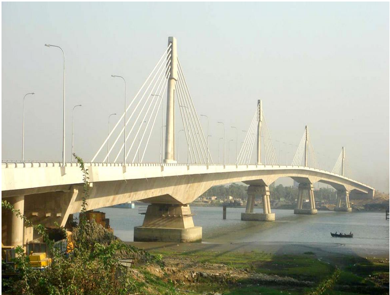
Figure 2.1: Cable Stayed Bridge, Shah Amanat, Chittagong
