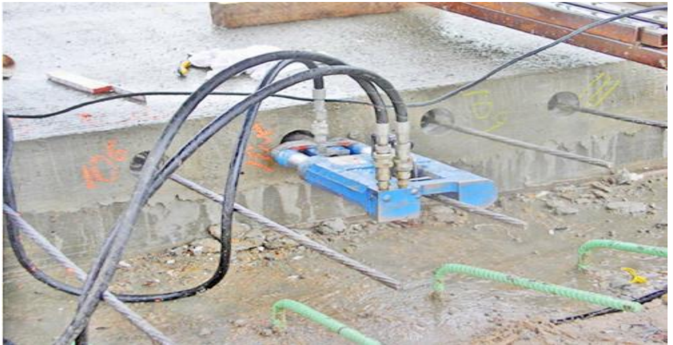
Figure 2.24: Post-tensioning Process
