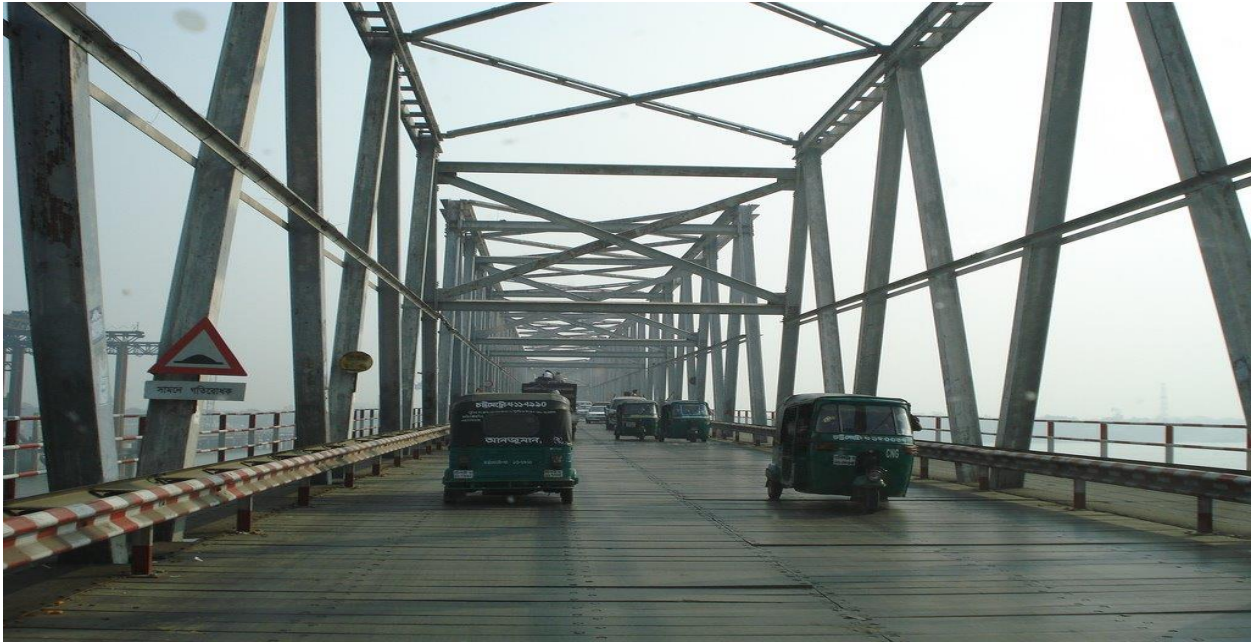
Figure 2.13: Truss with Timber Decks, Shah Amanat Bridge, Chittagong
