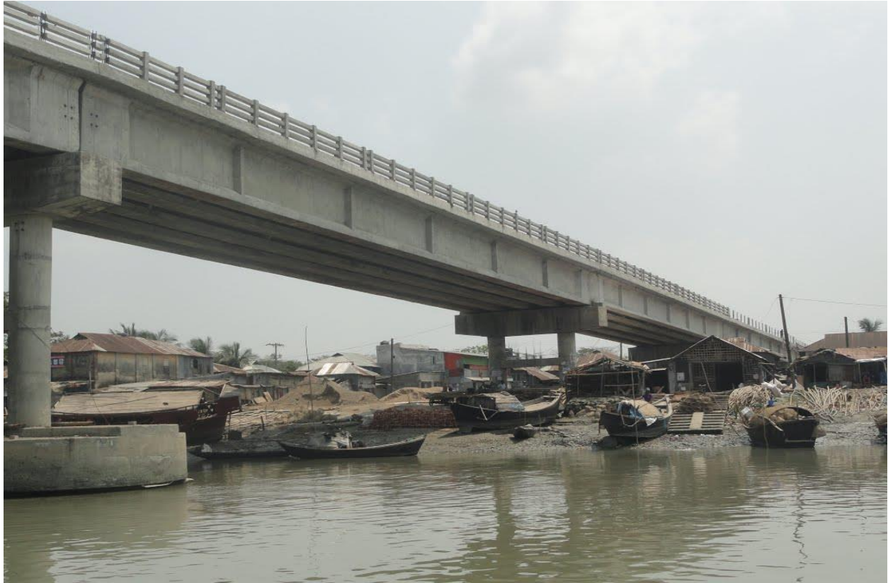
Figure 2.8: Pre-stressed Concrete (PC) Girder Bridge, Mohipur-Alipur, Patuakhali
