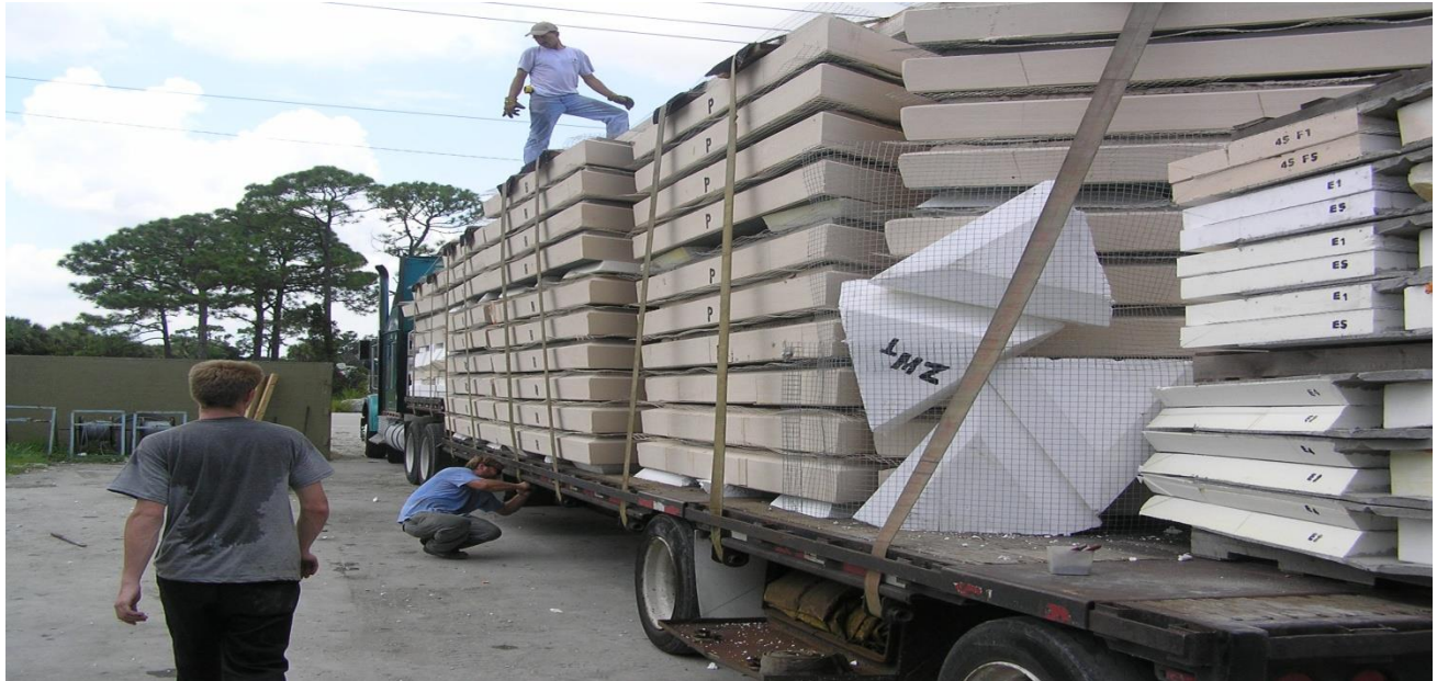
Figure 3.12: Transportation of Deck Panels
