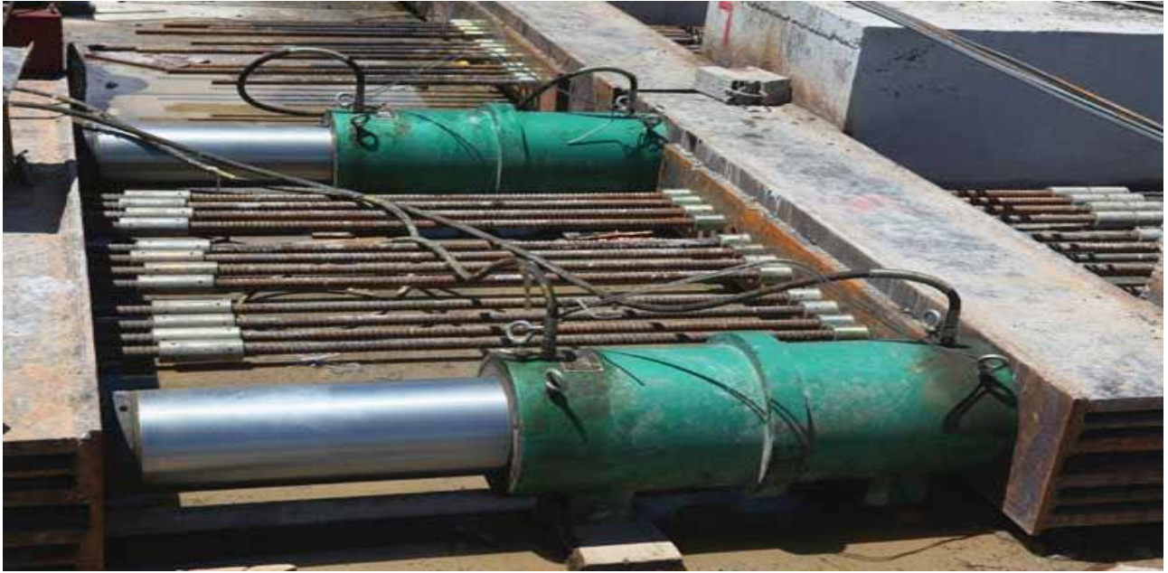
Figure 2.23: Pre-tensioning Process
