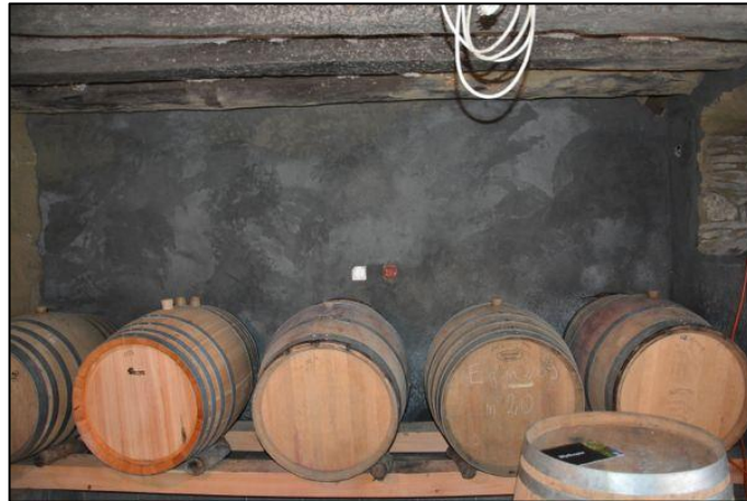
Fig 2.6: Biochar-Clay plaster in wine cellar
