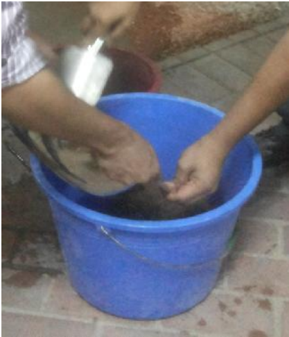
Figure A3 :- Material preparation for casting
